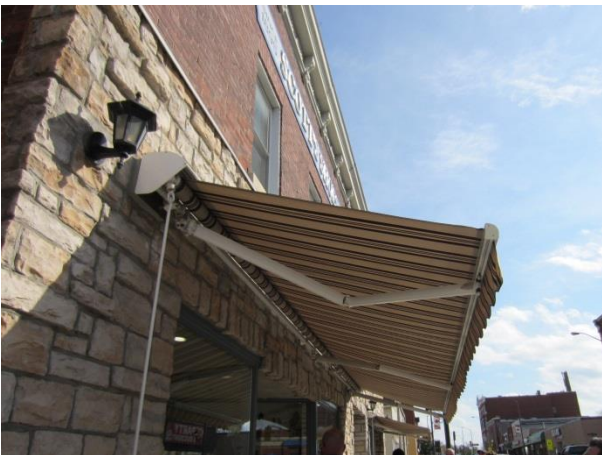
Awnings should be retractable, fabric and be suitable to provide shelter from the elements for pedestrians.
