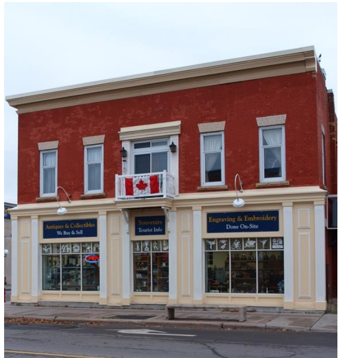
Signage should be incorporated into the storefront cornice or signboard where possible (example from Arnprior, Ontario).
