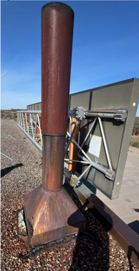
Figure 6 – Roof Vent Stack
