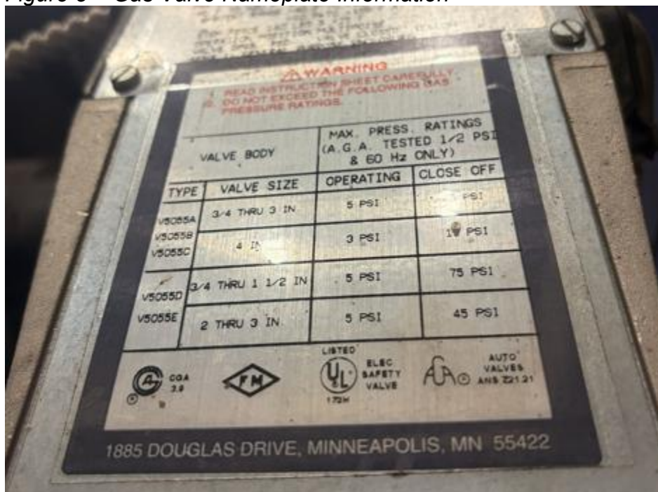
Figure 5 – Gas Valve Nameplate Information
