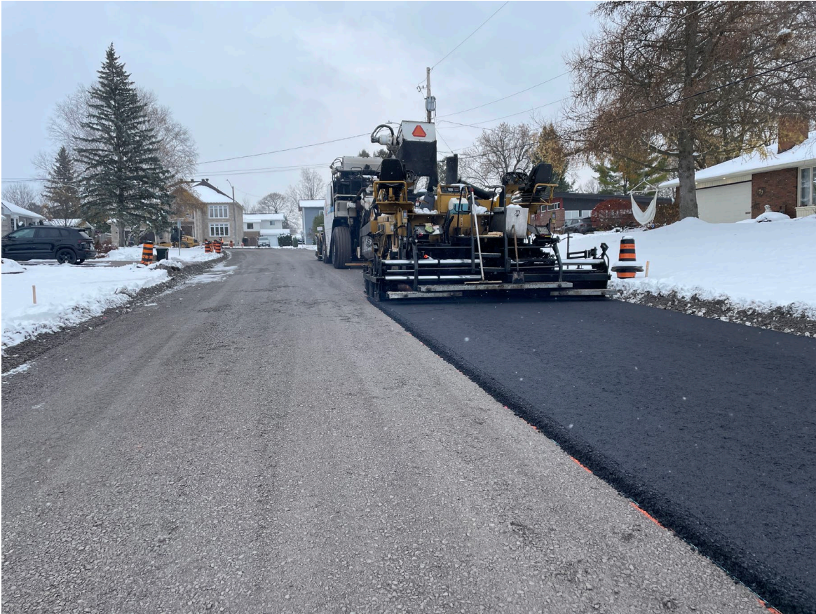
Completion of Stevenson Crescent base lift paving.
